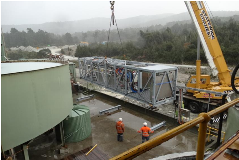
Figure 14: Synergen pilot plant being lowered into position at Henty Gold Mine in Tasmania
